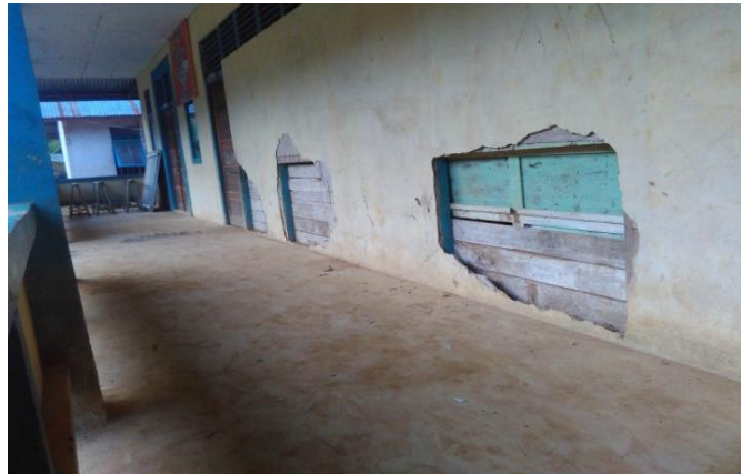
Figure 1. The Perforated Classroom Wall at SDN 14 Badat, Entikong District
