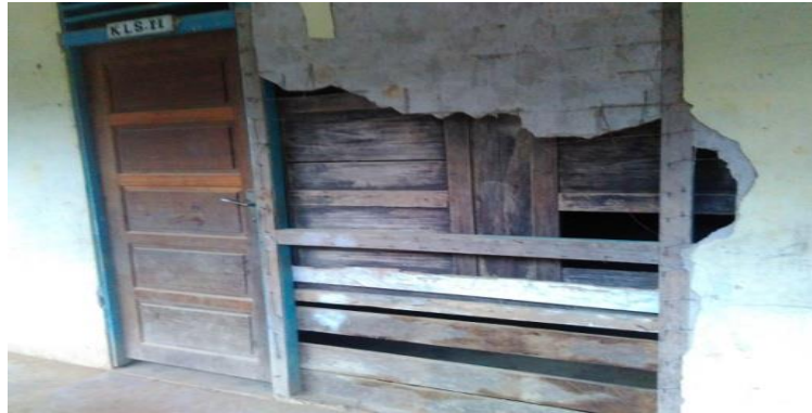
Figure 4. The Damaged Classroom Sills at SDN 28 Entabai, Sekayam District
