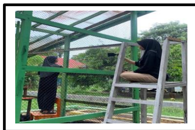
Gambar 3. Pengecatan Green House
