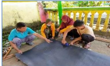
*Gambar 4. Pemasangan Dinding Greenhouse*
